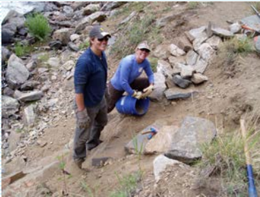
Volunteers repairing rock steps on a project in Clear Creek.
